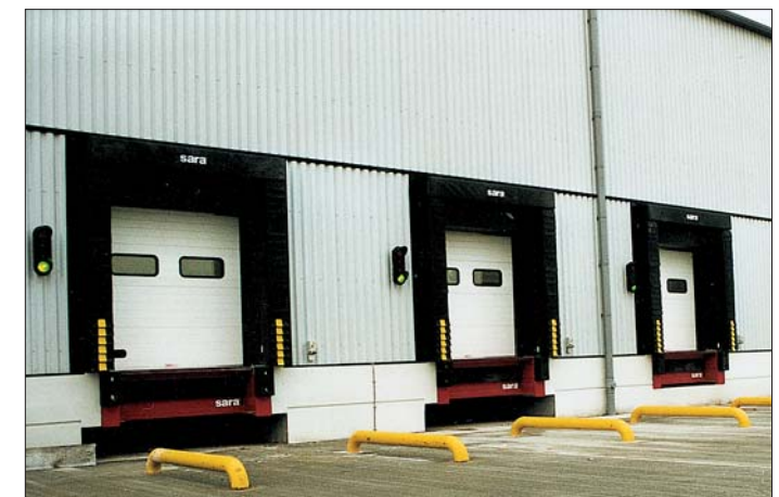
Loading Bays with 'Open Pit'
