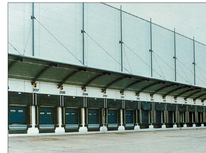
sara Pre-cast Concrete loading bay installation
