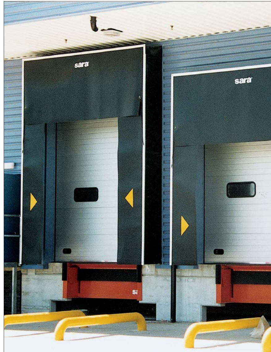
Telescopic Levellers with opening for vehicle tail lifts
