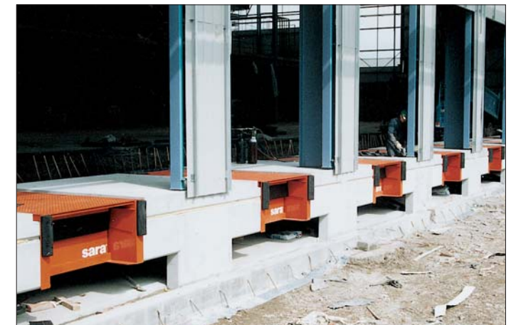
sara Levellers being set in sara Pre-cast Concrete Pits
