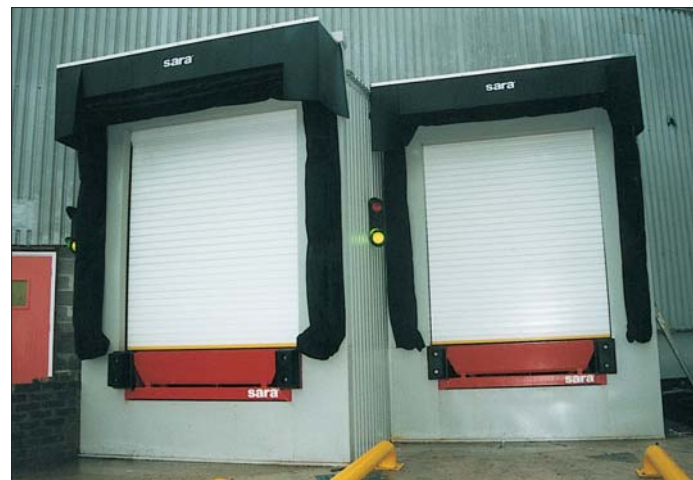
Levellers in factory extension (twin dock house)
