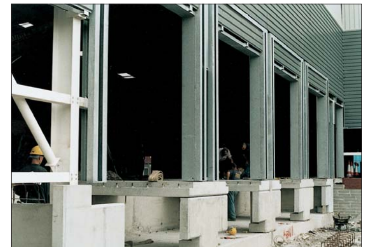
sara Pre-cast Concrete loading bay installation
